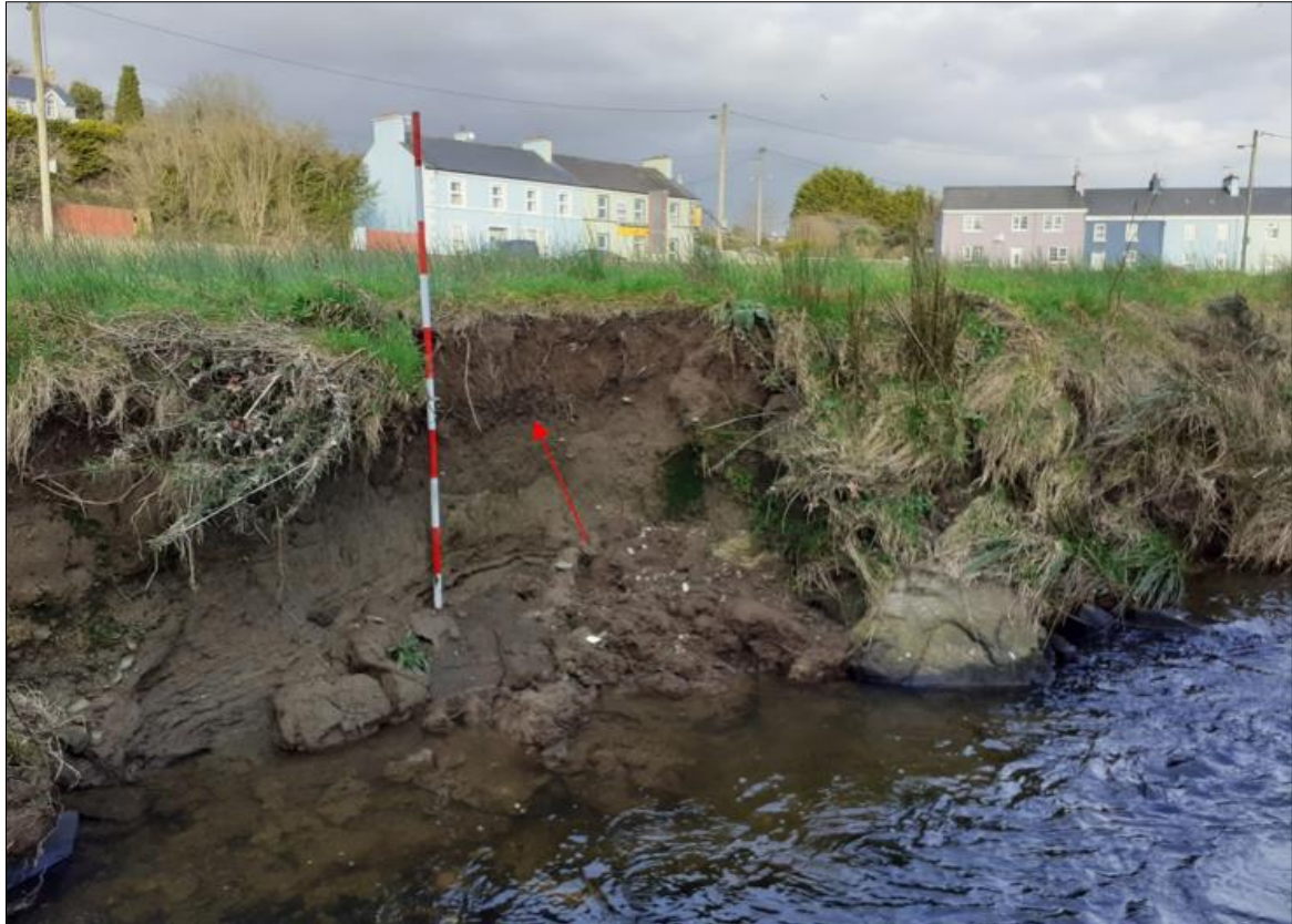
Figure 5: Location of exposed section of riverbank c. 105m downstream from proposed replacement bridge location
