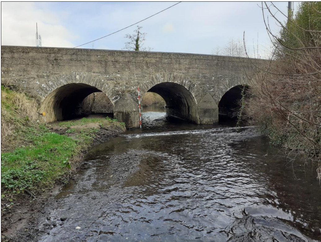
Plate 4: West (downstream) elevation of Burnfoot Bridge, facing east
