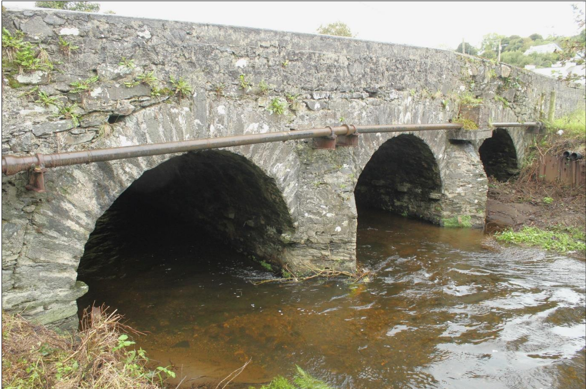
Plate 7: Original east elevation from south bank with segmental stone arches and triangular cutwaters. Keystone to voussoirs projects above arch extrados and arch barrel springs from course of projecting stones. Note partially-blocked northern archway and steel piles to both river banks.
