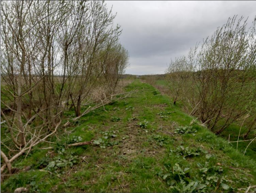
Plate 15.31: View towards west along Skeoge (northern) Embankment.
