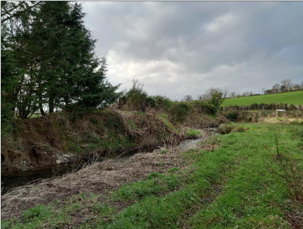
Plate 15.5: View to west along southern riverbank and existing earthen embankment area
