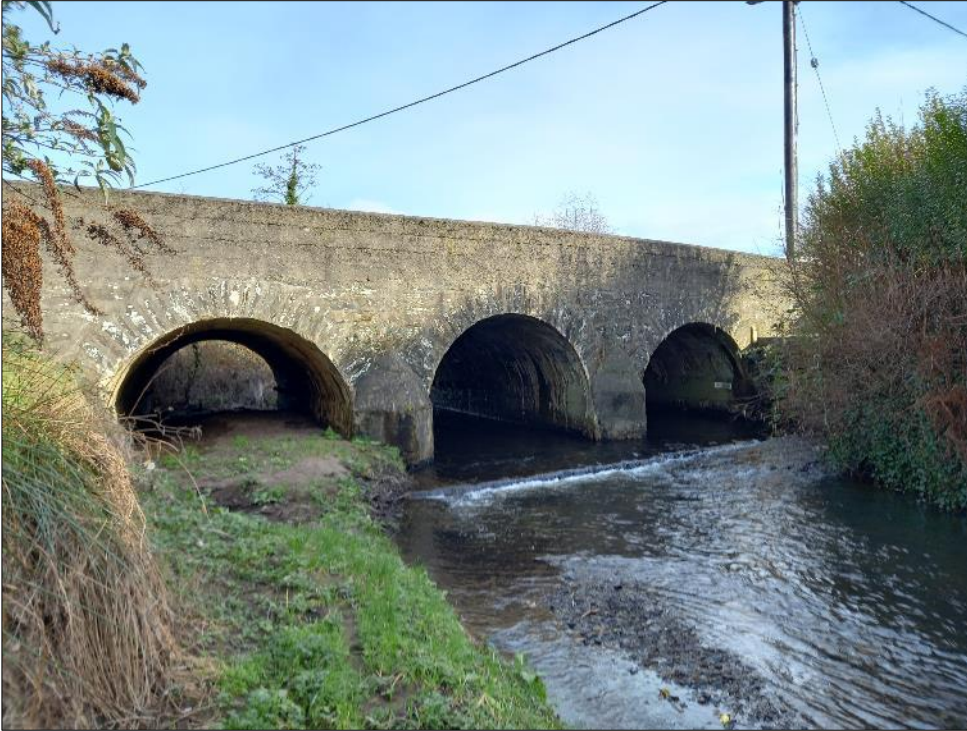
Plate 15.11: View towards east of western elevation of Burnfoot Bridge
