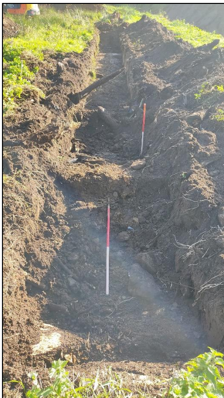
Plate 2: View of trench T1 (tree trunks) facing southwest
