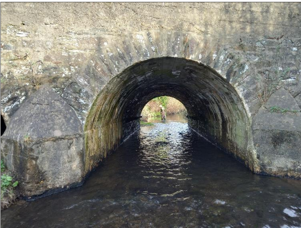
Plate 15.14: View towards east of central arch on western elevation. Note bridge widening represented by shuttered concrete soffit and concrete rendered cutwaters
