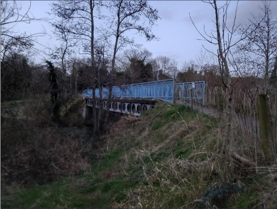
Plate 15.29: View towards northwest and pedestrian bridge at former Tooban Junction. This bridge forms part of the Inch Wildfowl Reserve walking trail
