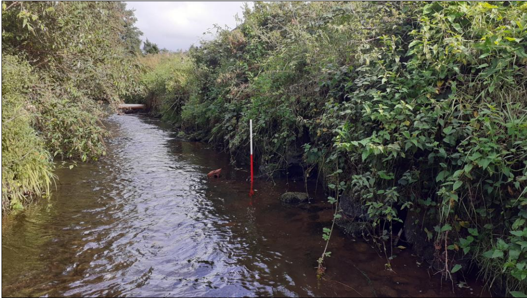
Plate 9: View of river channel facing east-northeast (approximately 100m upstream of Burnfoot Bridge). Note continued flood protection boulders and outflow pipe associated with Lios na Greine housing development
