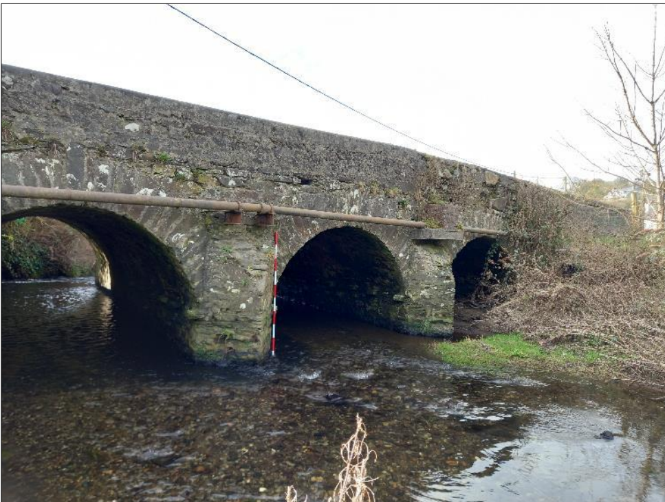
Plate 15.10: View towards northwest of eastern elevation of Burnfoot Bridge
