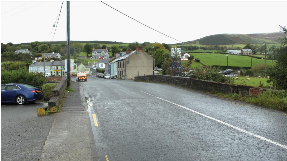
Plate 1: View to north over Burnfoot Bridge which carries R238 over Burnfoot River. Compare with historic photograph in Figure 3 (main text) which shows similar view prior to mid twentieth-century widening of bridge to west (left side of photograph) and levelling of roadway to reduce hump-back nature of crossing.
