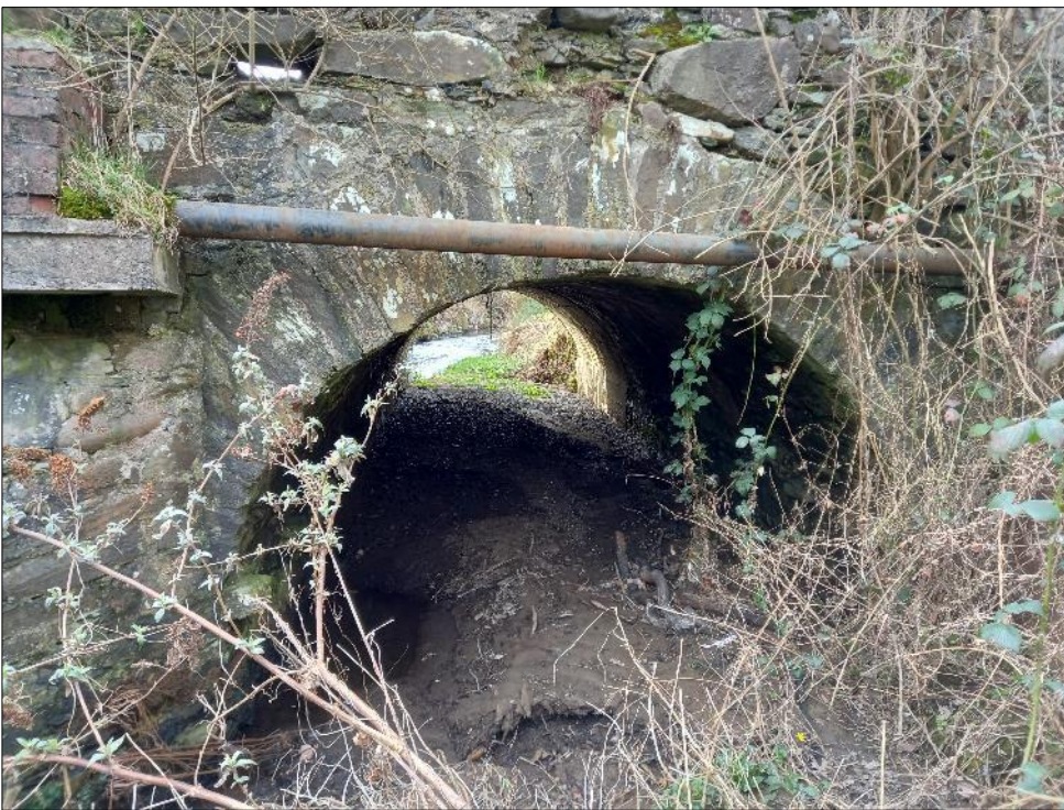
Plate 15.12: View towards west of northern silted bridge arch on eastern bridge elevation
