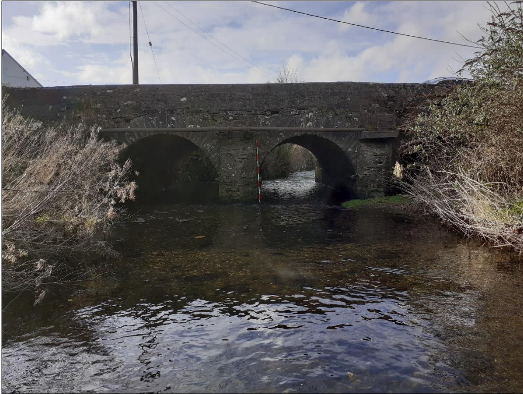
Plate 1: East (upstream) elevation of Burnfoot Bridge, facing west
