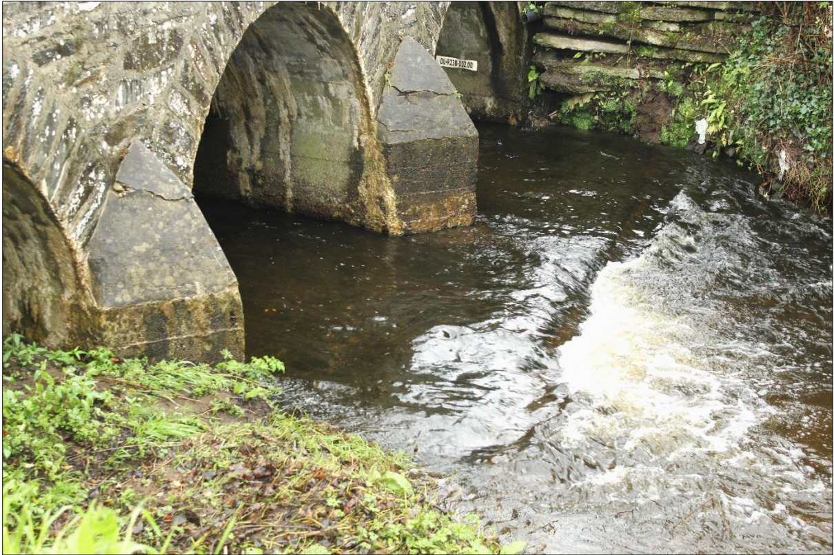
Plate 5: Detail of cast-concrete arch barrel and cutwater on west elevation.
