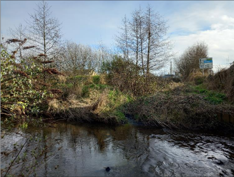
Plate 15.1: View towards southern riverbank at east side of Burnfoot bridge. Note disturbed ground and heavy vegetation
